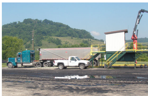
Coal weighing and sampling at Big Sandy coal wharf
