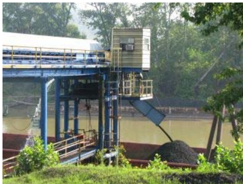
Barge loading at Wharf
