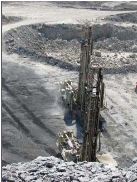
Overburden drilling at Tarkiln
